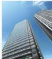
BRANZ TOWER WELLLITH SHINSAI-BASI II
