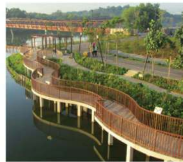
PUNGGOL WATERWAY, SINGAPORE
